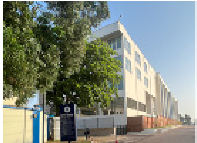
Supply and installation of air-condition units for Lincoln Community School's redevelopment Project Phase 1
