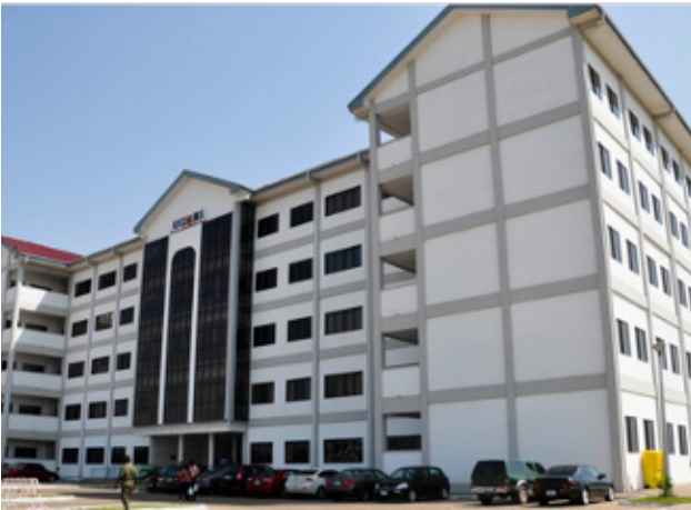
Supply and installation of VRF air-conditioners for KNUST Business School Phase 1
