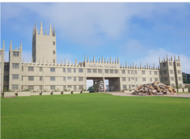
Supply of air-condition units for the Anagkazo Bible and Ministry Training College, Light House Chapel
