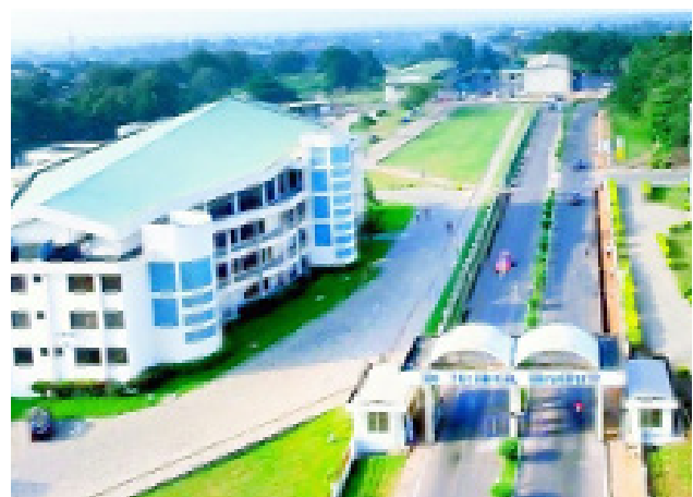
Supply and installation of split AC units for Ho Technical University
